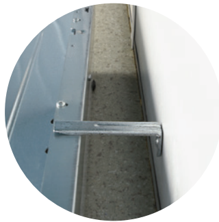
Wall Type Anti-Tip Bracket
